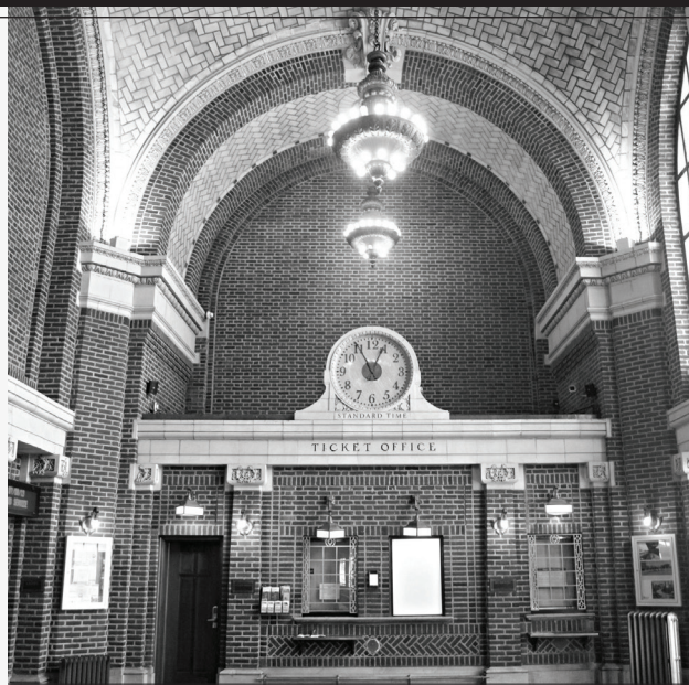
Today, Yonkers train station has features also found in Grand Central Terminal, including triangular lamps over the ticket booths and a vaulted Guastavino tile ceiling.
