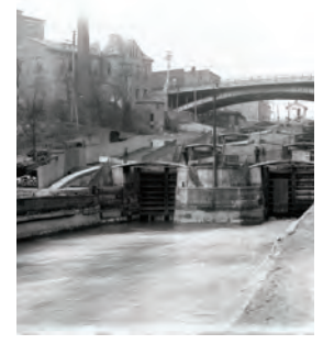
Enlarged Lockport "Flight of 5" twin staircase locks, April 8, 1907.
